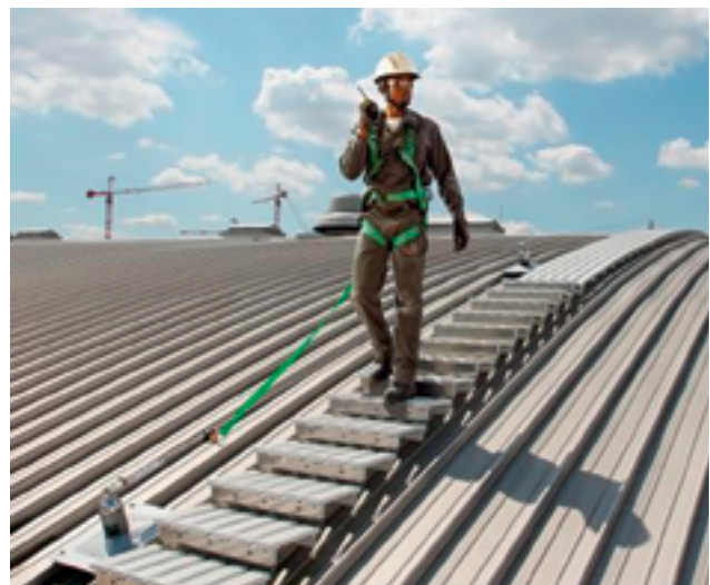
Figure 16 Work-restraint harness used during short-term inspection on a roof (image courtesy of MSA Safety)
