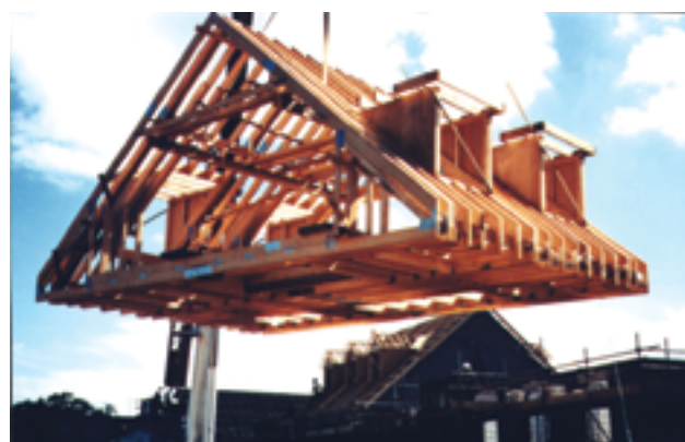
Figure 21 Craning a pre-assembled roof into position greatly reduces the need for work at height (image courtesy of the Trussed Rafter Association)
