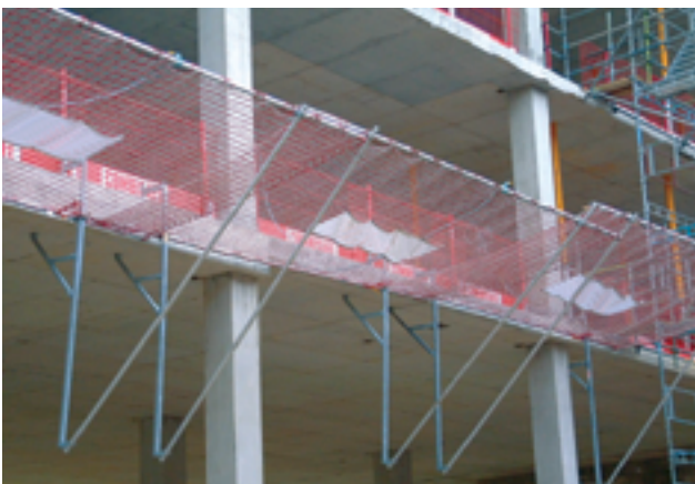
Figure 34(a) Debris netting (image courtesy of Combisafe)
