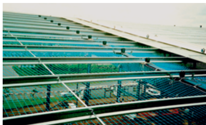
Figure 33 Use of safety nets during industrial roof work
