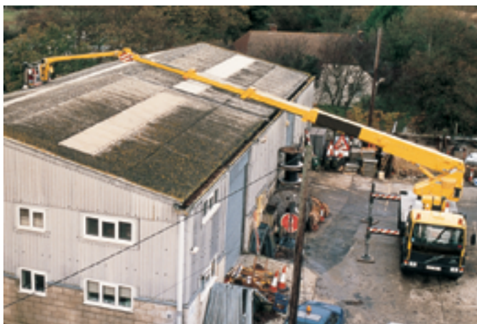
Figure 11 Powered access for inspecting a large fragile roof
