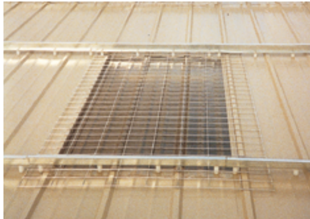
Figure 42 Galvanised mesh reinforcement between sheets of twin-skin roof light
