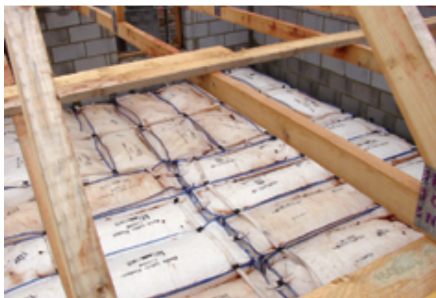
Figure 14(c) Beanbags being used as a fall mitigation measure during roof work (image courtesy of Forest Safety Products Ltd)
